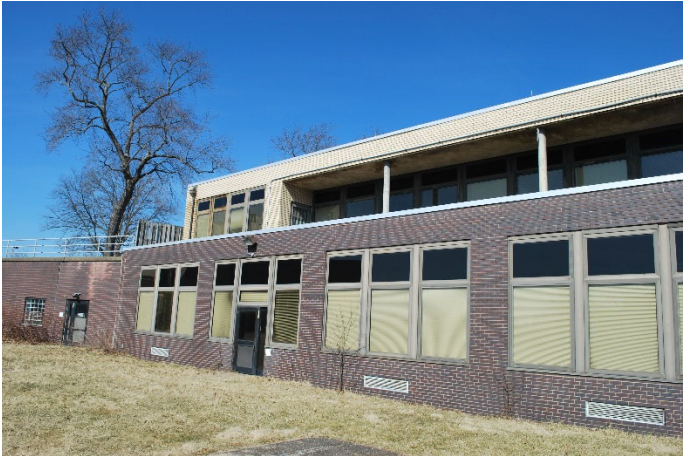
South Façade Detail
