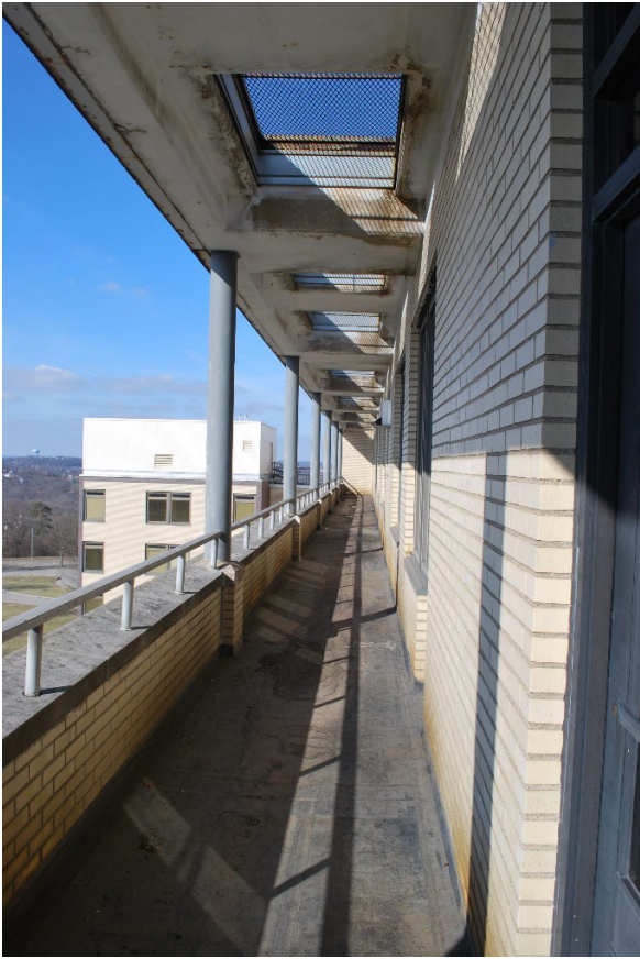
Sixth Floor Balcony
