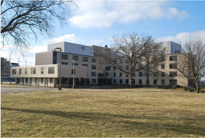
Entrance – Looking South
