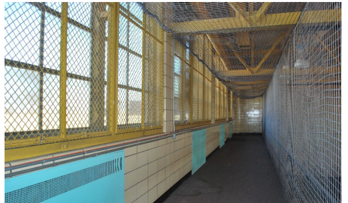
Gym Windows at Catwalk
