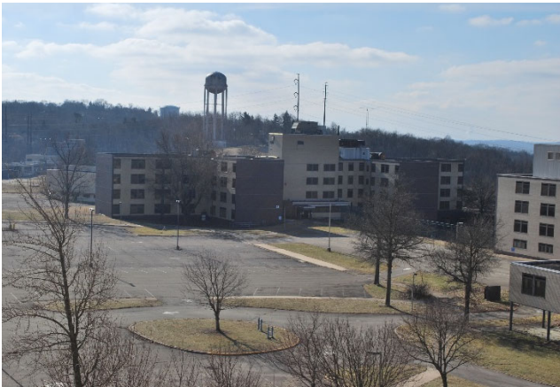
Looking Southeast from 6 th floor of Bldg. #1
