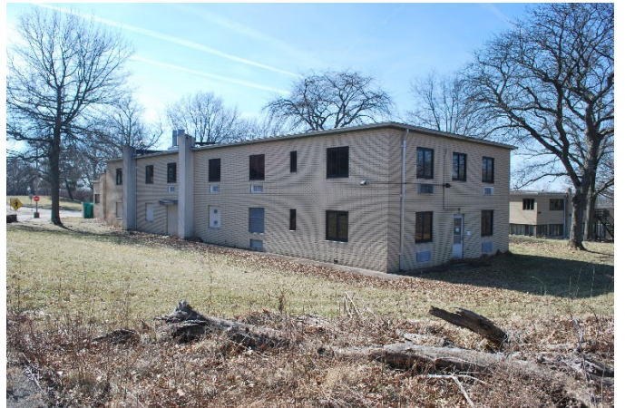
Building 13 Northeast Corner
