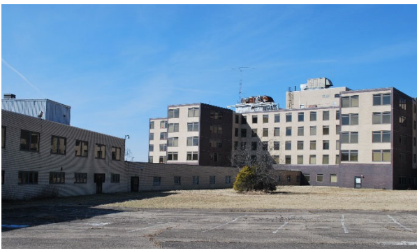
Buildings 4 and 8 looking East
