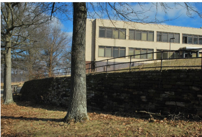
West Retaining Wall
