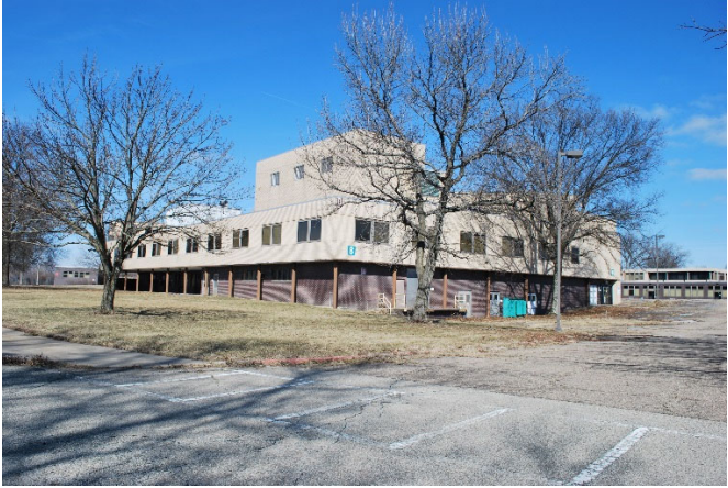
Southeast Corner from Bldg. 9 (fly loft)
