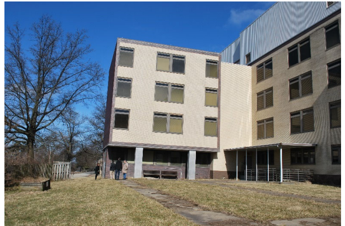
Rear Pavilion looking Northwest
