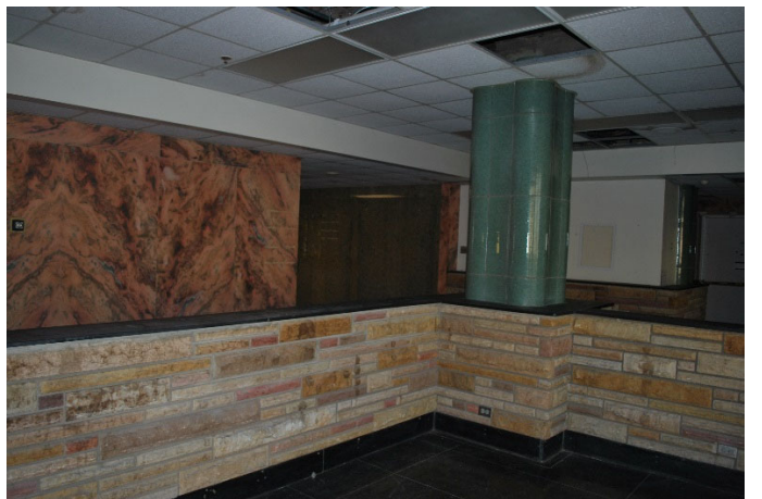
Lobby Column Cover and Marble
