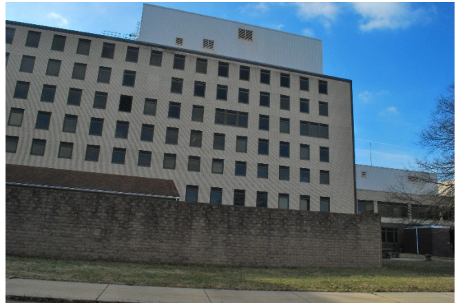
North Façade Looking South
