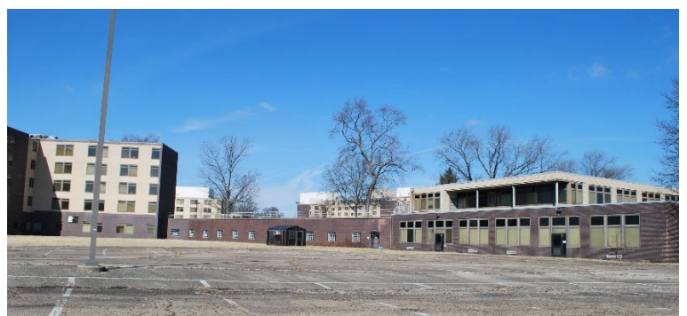
Buildings 4 and 7 looking North (Building 1 & 2 behind)
