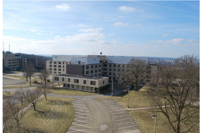
Looking South from 6 th Floor of Bldg. #1
