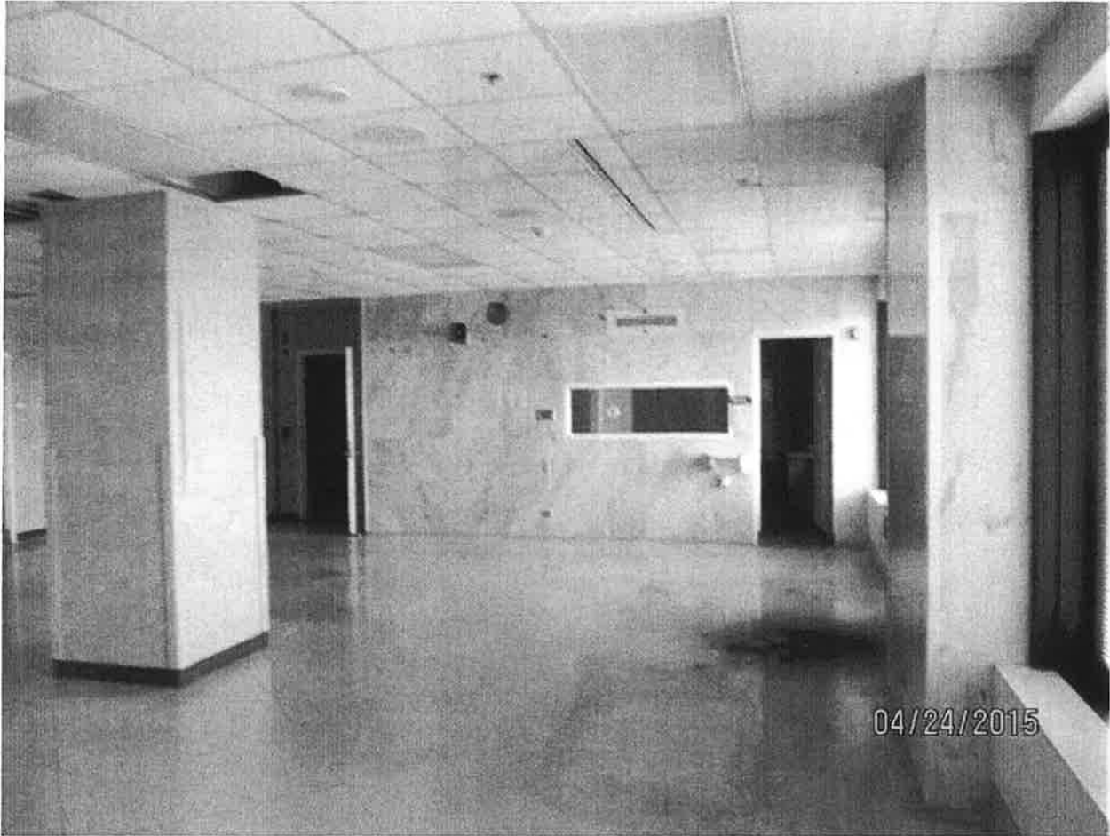
Photo taken in 2015 showing the remnants of the northwestern portion of the main lobby in Building 1. Behind the photographer in this view is a long corridor connecting this western half of the building to the eastern half. The northern wall is sheathed in marble.
