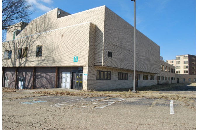
Northeast Corner with Bldg. 4 in background
