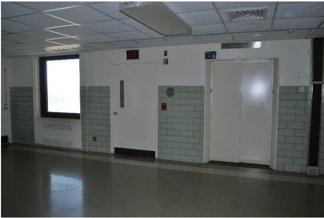
Fifth Floor Elevator Lobby
