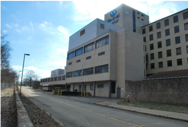
North Façade Looking East
